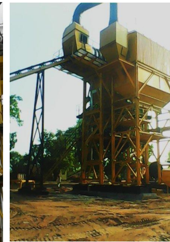
MSD 2000 Barbrik Projects Ltd Chhattisgarh
